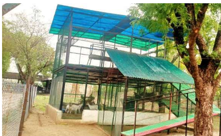
Fig. 4. Plastic based composite multi-purpose animal structure
